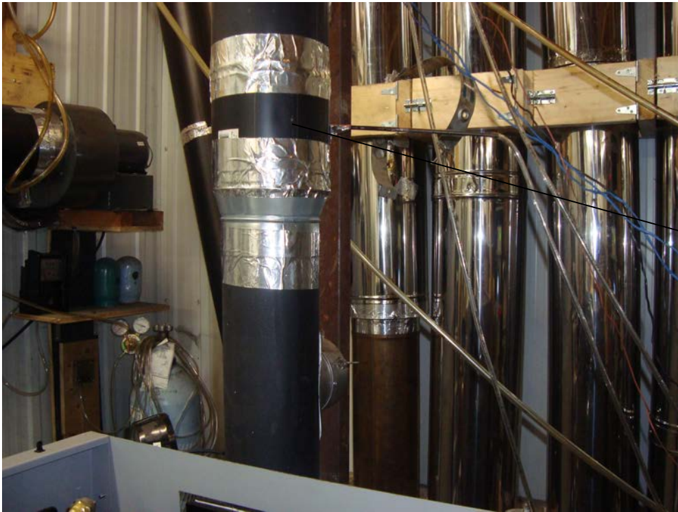
Draft Sampling port located 6in. From the flue outlet
